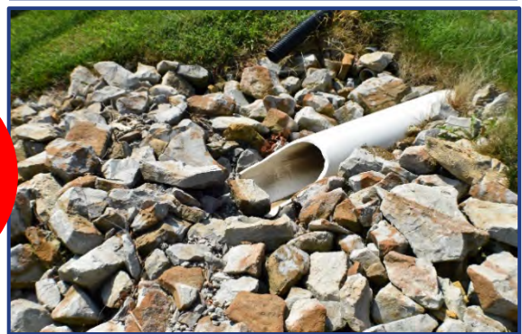
Pipe Condition AFTER Repair* (different diameter, material, installation)
