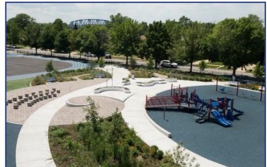
Left: Concrete curbs limit intrusions, while pea gravel prevents soil erosion within bioretention BMPs located on a downtown sidewalk. Source: City of Indianapolis IN. Right: Seating, permeable walkways, hardy shrubs, and a playset keep people out of a Chicago schoolyard’s bioretention BMP. Source: centerforgreenschools.org.
