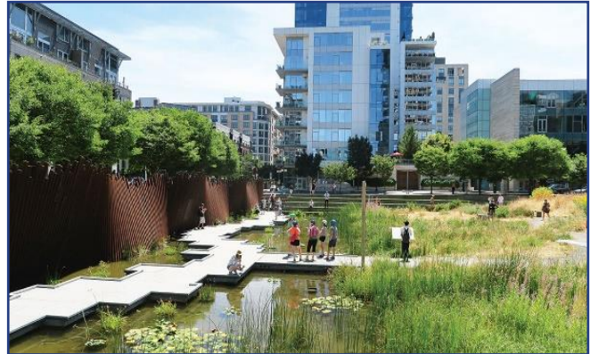
Above: A walkway allows pedestrians to go into a stormwater wetland BMP. Source: City of Portland, OR
