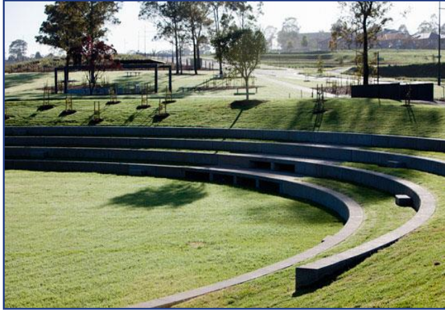
Left: A detention BMP also functions as an amphitheater, ensuring its maintenance, and giving it a neat and tidy appearance. Source: City of Philadelphia PA ; Right: Experienced landscape professionals can make a detention basin an attractive landscape feature. Source: Urban Drainage and Flood Control District Manual, Volume 2.
