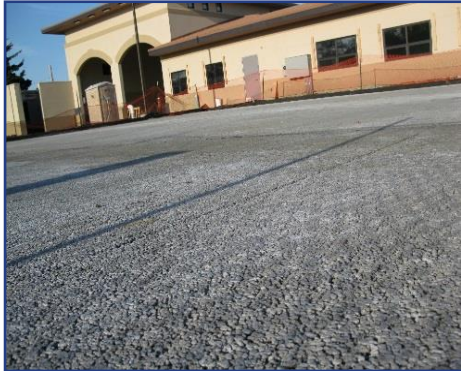
Above: Pervious concrete requires minimal routine maintenance. Source: City of Lenexa KS Fire Station #5; Right – Source: Kansas City Zoo
