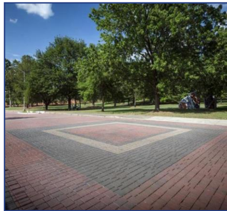
Left: Permeable pavers create a decorative, functional parking lot located on a large corporate campus in Indianapolis IN. Source: Heather Williams, LEED-AP. Middle and Right: Different colors, patterns, and configurations of permeable pavements are used in urban Atlanta GA neighborhoods to manage local drainage and add to the character of the community. Source: City of Atlanta GA
