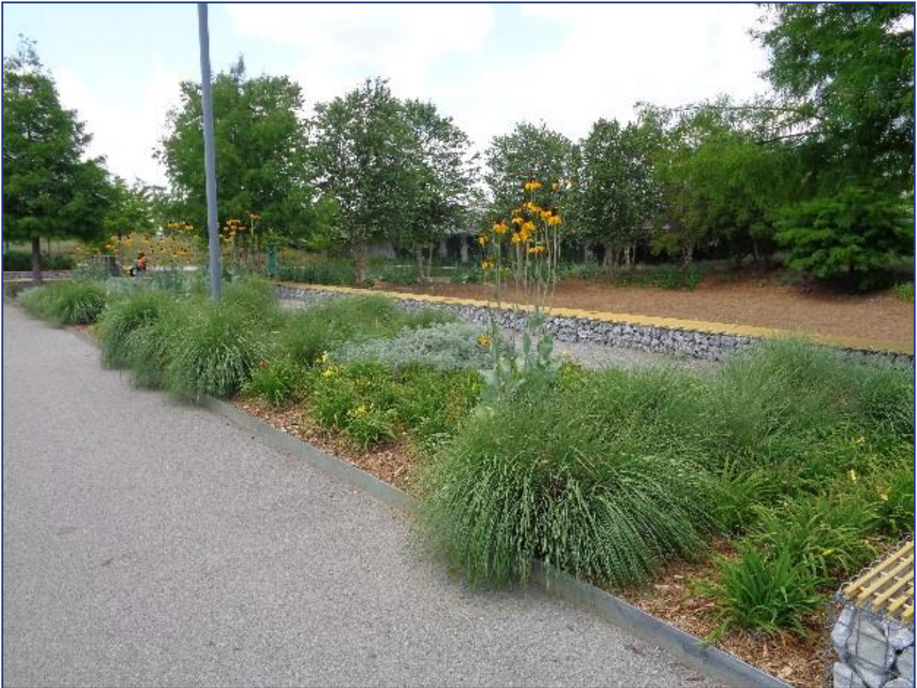
Figure 5-6. Bioretention BMP with a Pervious Concrete Apron
