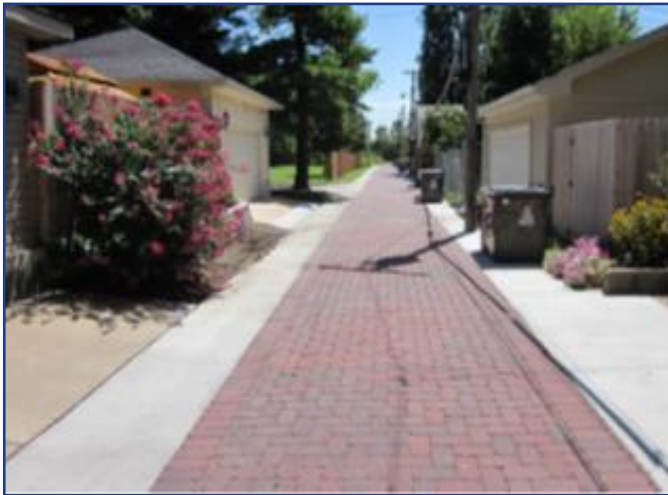
Left: Pervious pavements are not easily clogged by plant debris making them good choice to enhance urban and suburban landscapes. Source: St. Louis Metropolitan Sewer District. Above: In contrast, proprietary media filters, baffle boxes, and similar BMPs may become clogged quickly in these areas. Source: City of Maple Valley, WA.
