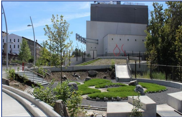
Above: Pathways along and through a bioretention BMP. Source: City of Philadelphia PA Water Dept.
