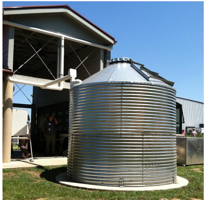
Above: Cistern used to capture overflow from a green roof for site irrigation is installed at the Kansas City Performing Arts Center garage. (Photo: Courtesy of Jeffrey L. Bruce & Co., Kansas City MO); Right: Cistern used for site irrigation at a Chattanooga Area Food Bank in Chattanooga, TN. (Photo: Wood E&IS)
