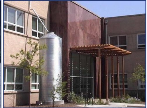
Above: Cisterns can be paired with irrigation systems for more sustainable maintenance practices. Source: Lake County, IL
