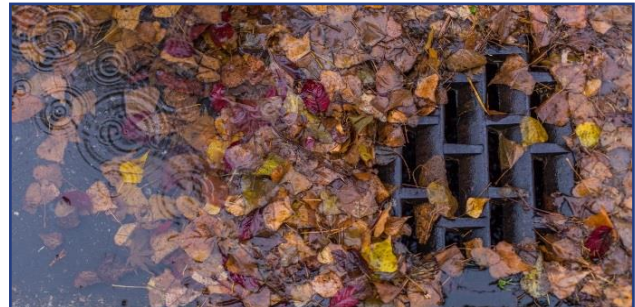
Left: Pervious pavements are not easily clogged by plant debris making them good choice to enhance urban and suburban landscapes. Source: St. Louis Metropolitan Sewer District. Above: In contrast, proprietary media filters, baffle boxes, and similar BMPs may become clogged quickly in these areas. Source: City of Maple Valley, WA.
