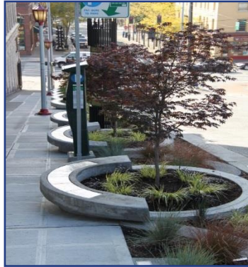
Figures 3-20a through d. Protecting BMPs with Hardscape Barriers
