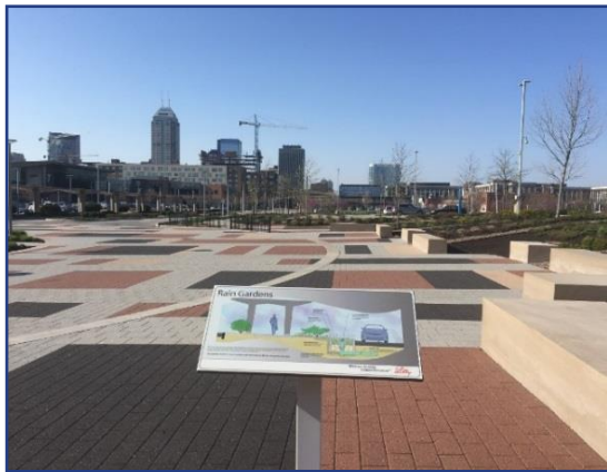
Left: Permeable pavers create a decorative, functional parking lot located on a large corporate campus in Indianapolis IN. Source: Heather Williams, LEED-AP. Middle and Right: Different colors, patterns, and configurations of permeable pavements are used in urban Atlanta GA neighborhoods to manage local drainage and add to the character of the community. Source: City of Atlanta GA
