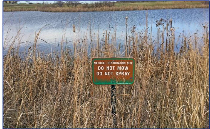
Left: Tall grass buffer help to create a “naturalized” stormwater pond that deters waterfowl residence. Source: Lake County, IL. Right: A “no mow” sign stands in a tall grass stormwater BMP buffer in Merrillville IN. Source: Municipal Sewer & Water Magazine.
