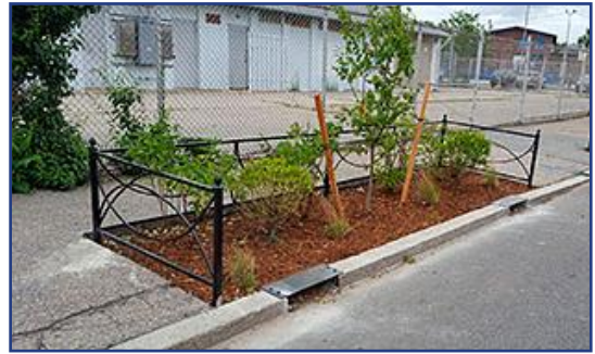
Figures 3-19a and b. BMP Fencing Examples
