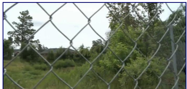
This fenced retention BMP is located behind a neighborhood, where it was not maintained. BMPs like this become an eyesore and source of complaints. Source: WRDW Augusta GA
