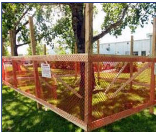
Figures 3-13a and b. Mature Tree Protection During Construction
