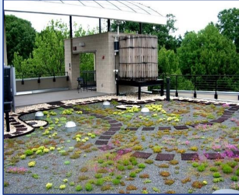
Cistern with overflow pipe to a green roof. Source: City of Atlanta GA
