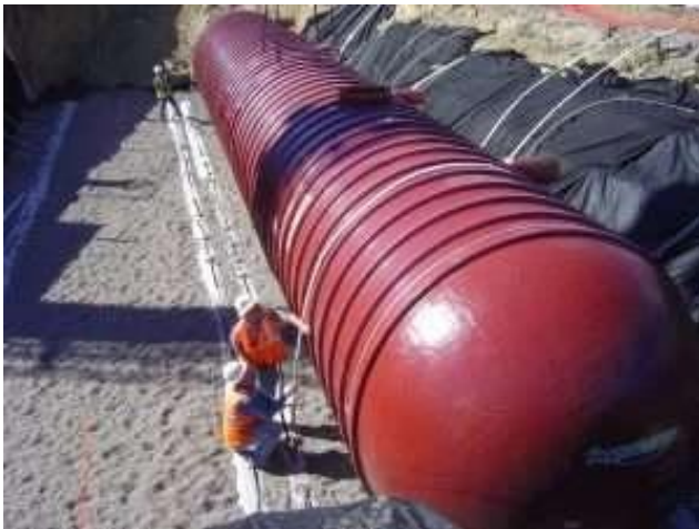
Above: Cistern used to capture overflow from a green roof for site irrigation is installed at the Kansas City Performing Arts Center garage. (Photo: Courtesy of Jeffrey L. Bruce & Co., Kansas City MO); Right: Cistern used for site irrigation at a Chattanooga Area Food Bank in Chattanooga, TN. (Photo: Wood E&IS)
