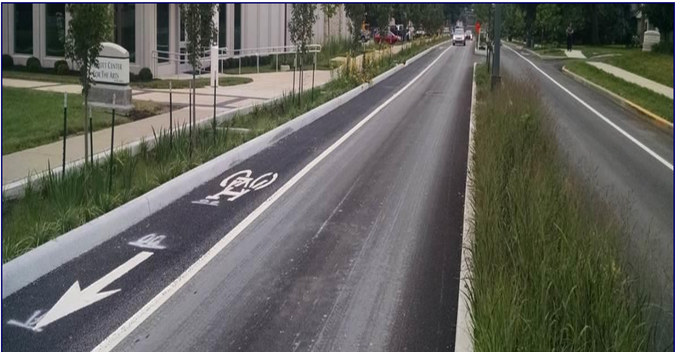
Green boulevard at Butler University in Indianapolis IN. Low-maintenance vegetated swales are used for landscaping and runoff conveyance. Bike lanes add a multi-modal element to the overall design. Source: Heather Williams LEED-AP
