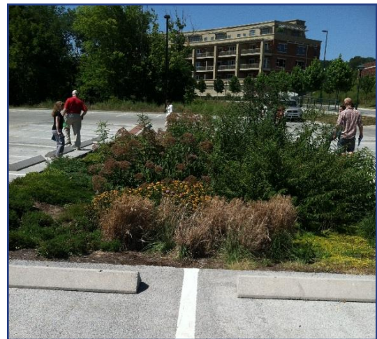
Above: Native bioretention BMP combined with permeable concrete in an urban bus stop parking area in Chattanooga, TN. Source: City of Chattanooga TN
