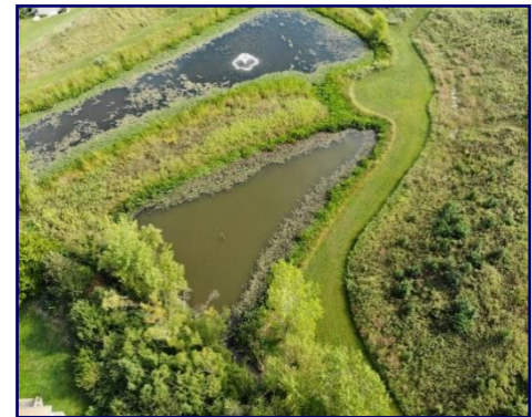
The mowed strip of land around these Topeka area retention BMPs indicate the location of the unobstructed access easement. Source: City of Topeka
