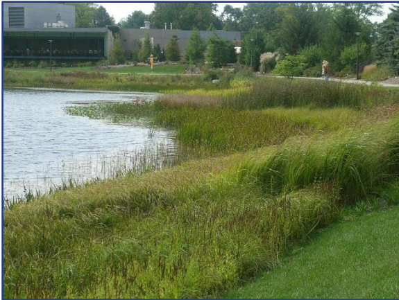
Left: Tall grass buffer help to create a “naturalized” stormwater pond that deters waterfowl residence. Source: Lake County, IL. Right: A “no mow” sign stands in a tall grass stormwater BMP buffer in Merrillville IN. Source: Municipal Sewer & Water Magazine.
