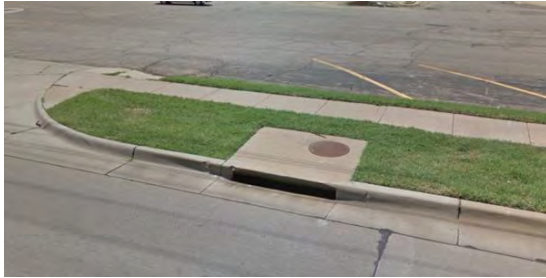
Example 1 Reconstruct street and add curb with enclosed storm system
