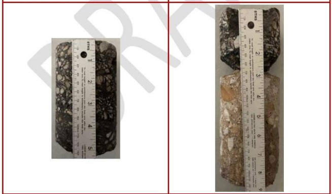
Photo #3: 5.25-inches asphalt
