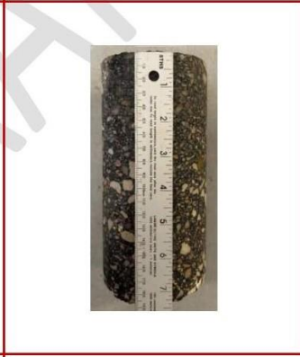
Photo #8: 7.5-inches asphalt
