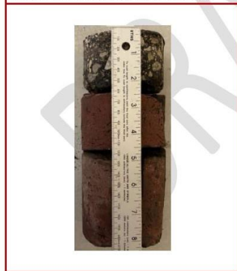
Photo #11: 2.5-inches asphalt, 5.75-inches Brick
