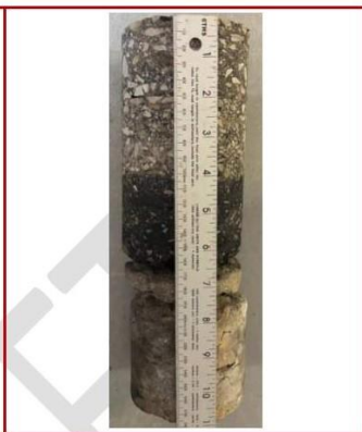
Photo #6: 6.5-inches asphalt, 4.5-inches concrete
