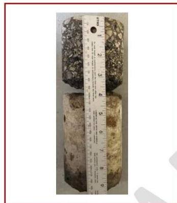
Photo #5: 3.75-inches asphalt, 5.5 concrete
