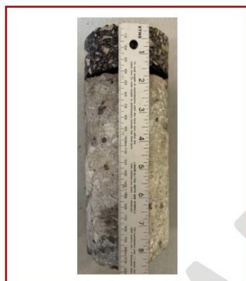
Photo #9: 1.5-inches asphalt, 7.25-inches concrete
