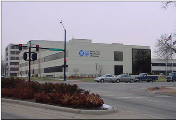
Blue Cross Blue Shield office building addition located at the intersection of SW 12 th and Topeka Blvd.
