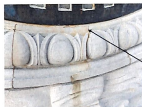
STONE INJECTION REPAIR D3 SCALE: NONE
