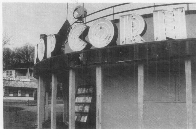
17. Glen Echo Park near Washington, D.C., is an early 20th century amusement park. (It is the home of the first bumper car ride in the world.) Its neon signs needed repair: (a) tubes were broken and the surrounding "metal cans" needed work also; (b) and (c) removal of the back of "Candy Corner" sign revealed debris from insects and birds; (d) preparing the "metal cans" from the "Pop Corn" sign for remounting; (e) and (f) neon fabricators installing the new tubing in the repaired and remounted cans; (g) repairs finished, the relit signs enliven the park once again. Photos: (a-c) Stan Fowler; (d-f) Larry Kanter; (g) Rebecca Hammel.
