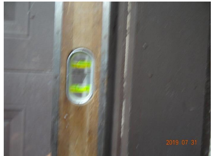
Fig. 8 Door out of plum
