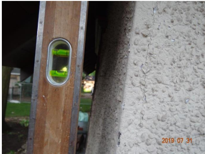
Fig. 7 Wall 2 ½" out of plum
