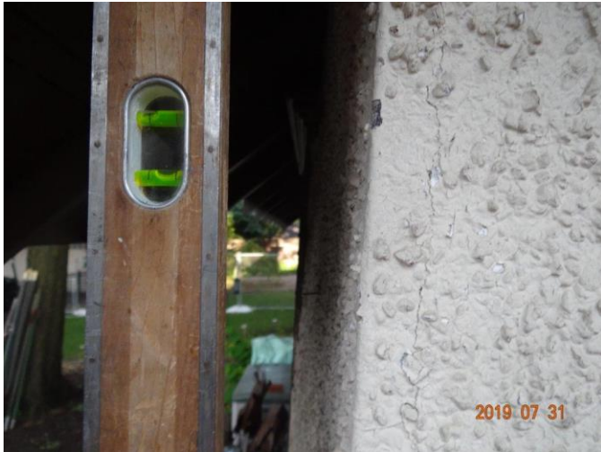
Fig. 5 Wall 2 ½" out of plum
