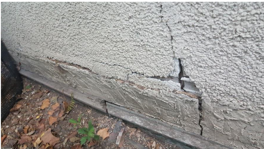
Fig. 1. Foundation (Top) Fig. 2. Door opening. (Left) Fig. 3. Trim detailing. (Right) Fig. 4. Stucco Crack (Bottom)
