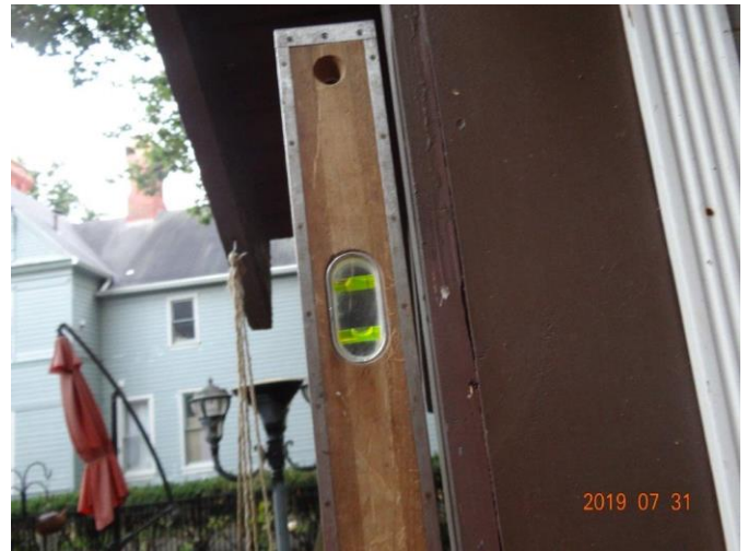
Fig. 6 Wall out of plum
