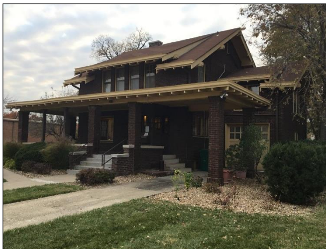
Figure 17. 1915 Craftsman/Bungalow; 835 SW Western Avenue; view facing west. Source: Stantec, 2021.
