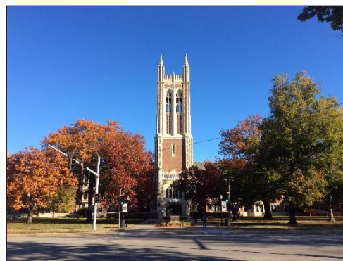
Figure 16. 1931 Collegiate Gothic style Topeka High School; 800 SW 10th St.; view facing north. Source: Stantec, 2021.
