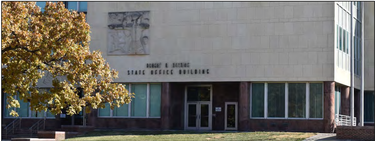
Photograph 29. Kansas State Office Building, red granite panels along ground floor and limestone panels on lower blocks
