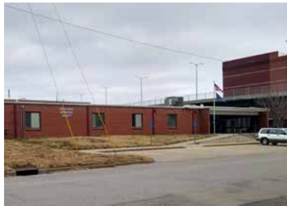
TMTA Facility, Image courtesy of Stantec
