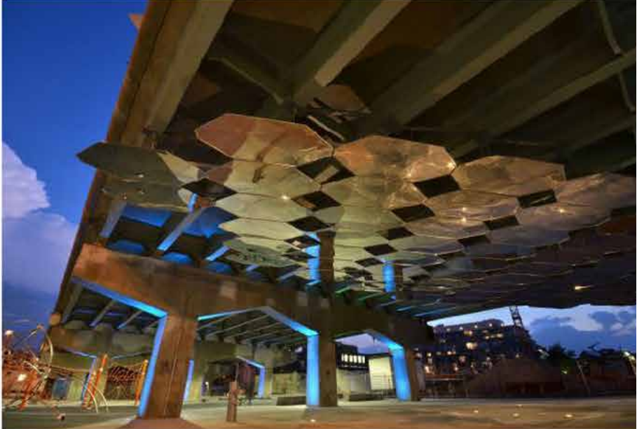
(above) Underpass Park, Toronto, Canada. Images courtesy of Stantec; (right) 14th Street Viaduct, Hoboken, NJ;
