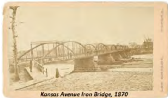
Kansas Avenue Iron Bridge, 1870
