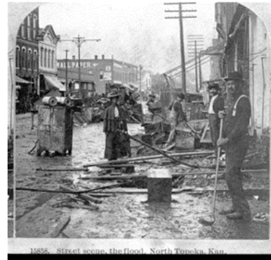
Flood damage along N. Kansas Ave., 1903
