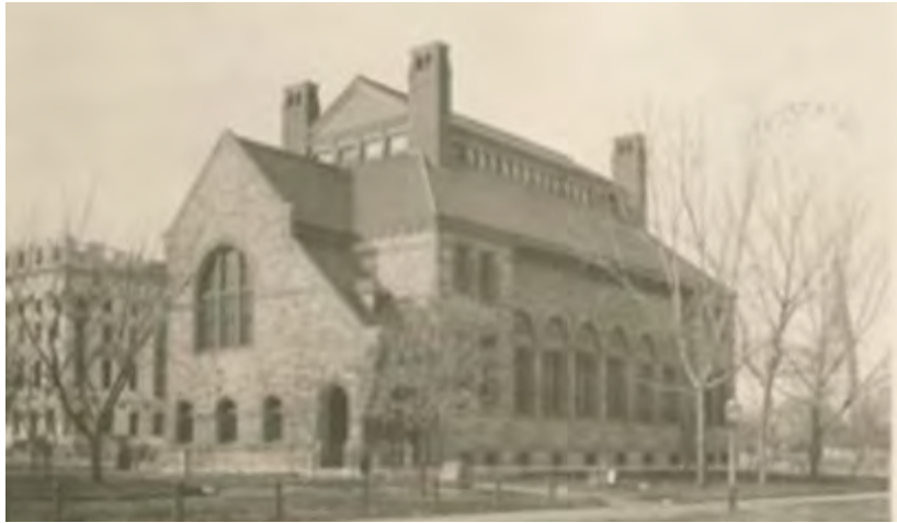
Topeka Free Public Library with the Kansas State Capitol under construction in the background, 1888
