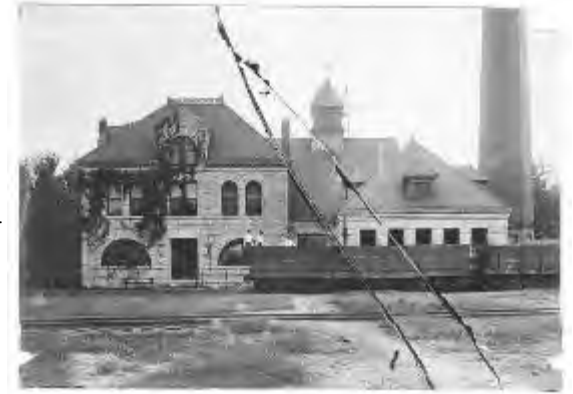
Topeka Municipal Water Works Plant SW Crane & Harrison St., circa 1895
