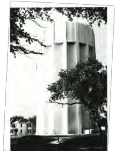
11th & Quincy Water Tower. 1943
