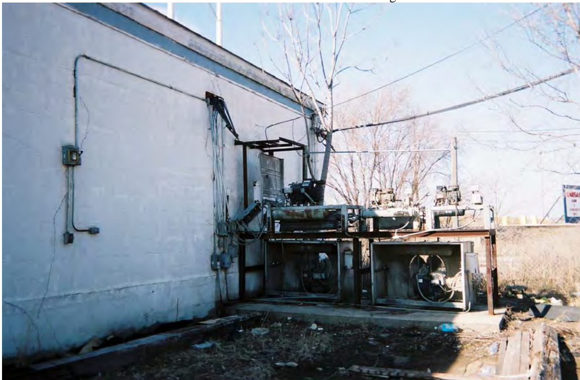
Photo 4 Former cooling equipment (abandoned) on the northwest corner of the building.
