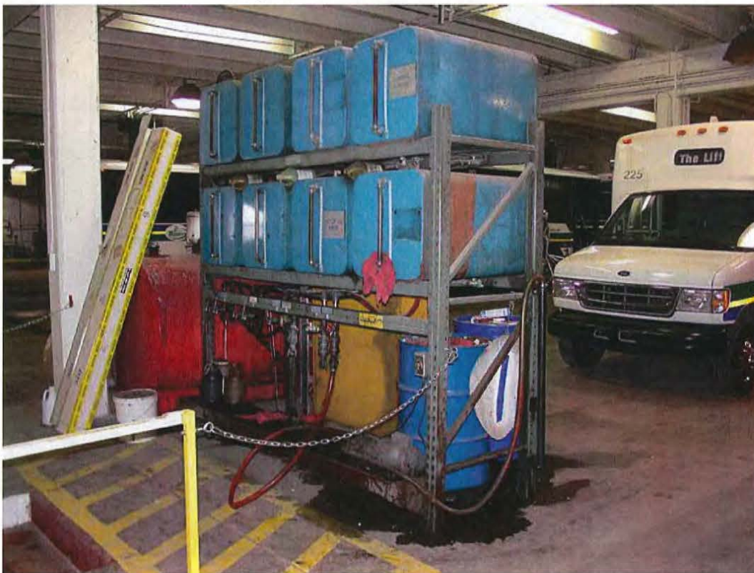
Photo 16 Oil storage area at TMTA's 201 N Kansas Ave building. A large oil stained area surrounds a portion of the storage shelf.
