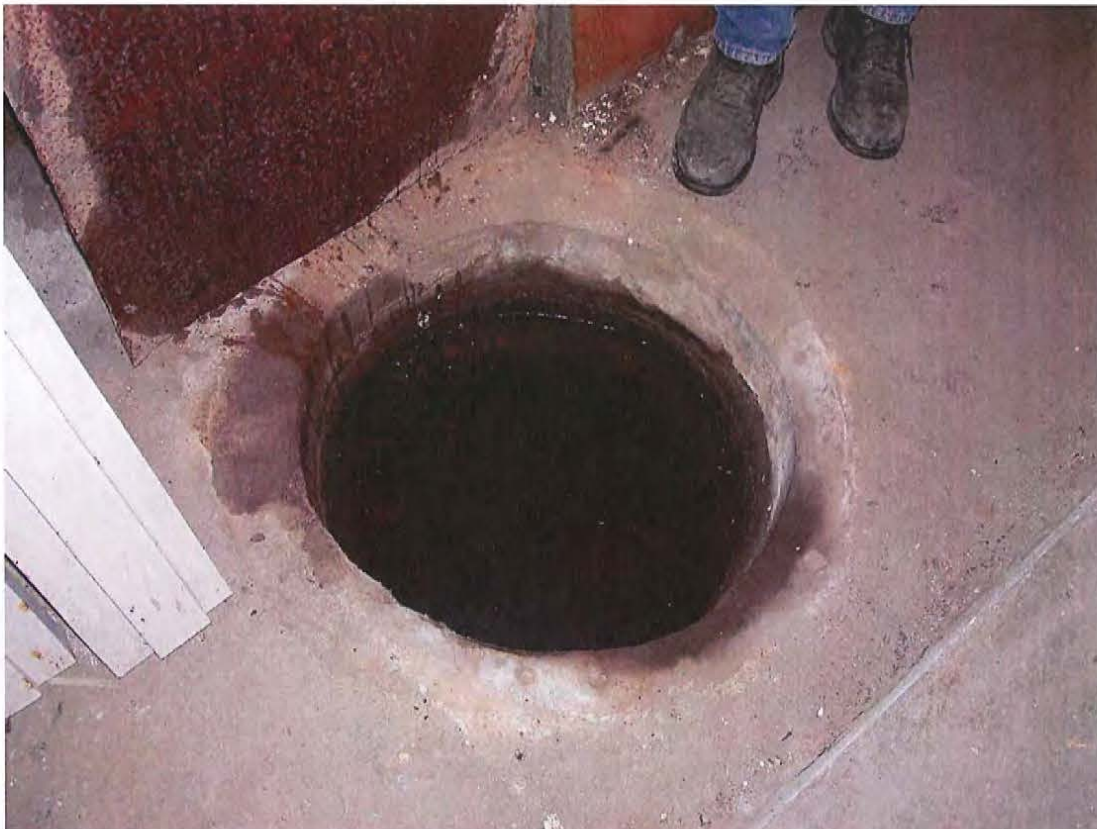
Photo 6 Sump in the basement of the building, usually covered by a metal plate.
