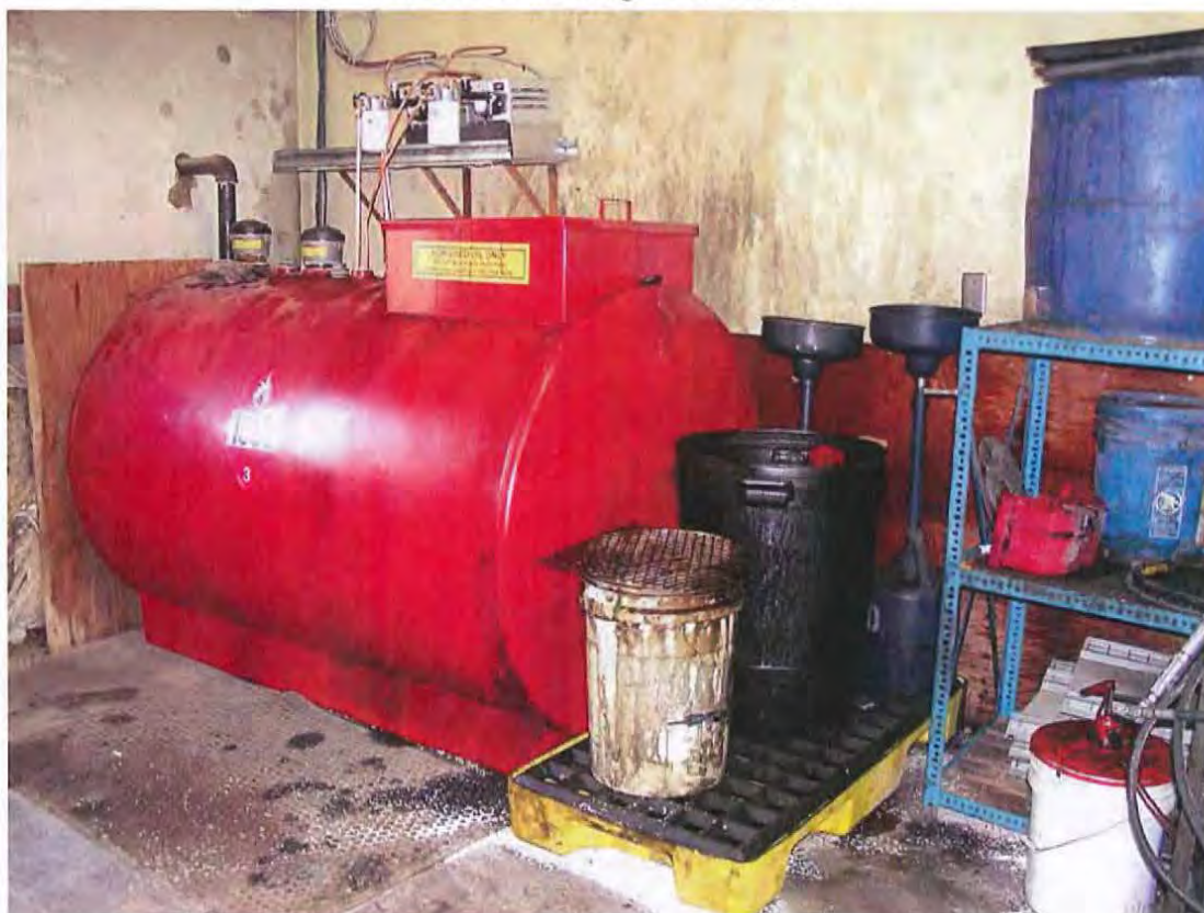
Photo 14 Used oil AST and drums in Fleet Services maintenance bay.
