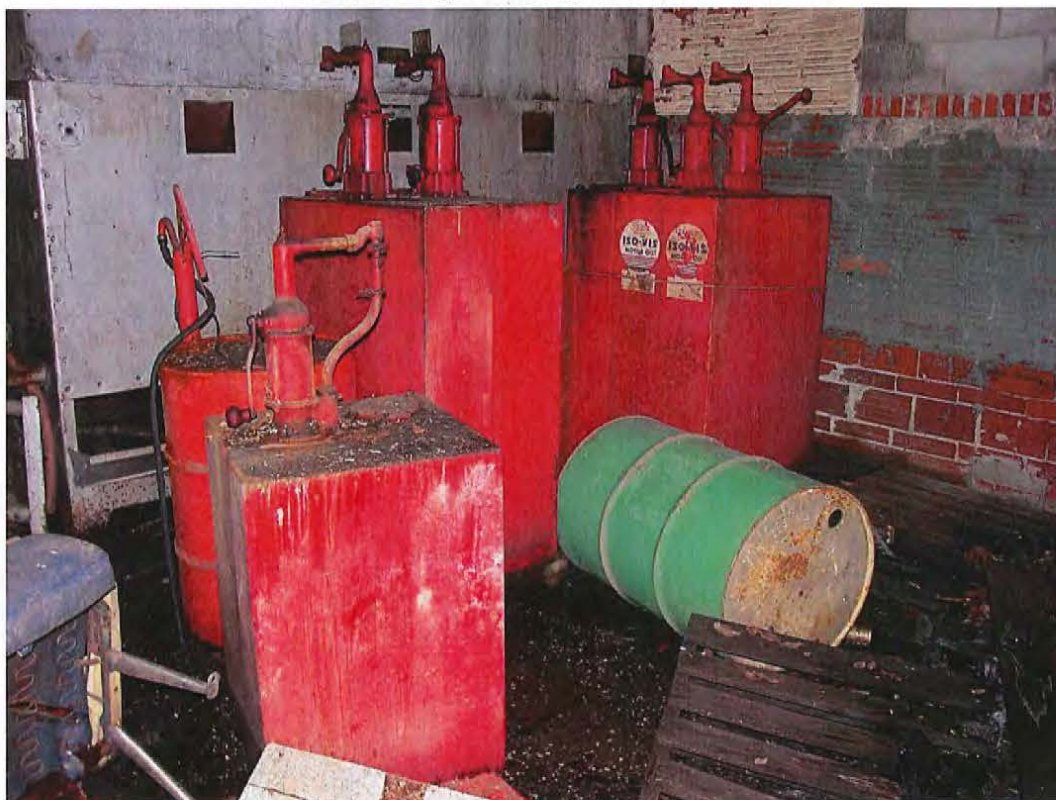
Photo 8 Drums and ASTs inside the former engine building, in the northern section. Some staining is visible at the base of the ASTs.
