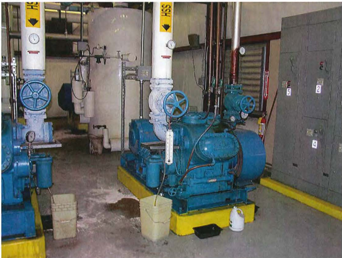
Photo 8 Engine room. Small stains are visible throughout the room. Oil dry is used to absorb the spills.
