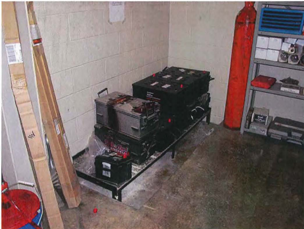
Photo 12 Battery storage area at TMTA's 200 NW Crane St. building. Battery storage containment drains to neutralizing UST located
