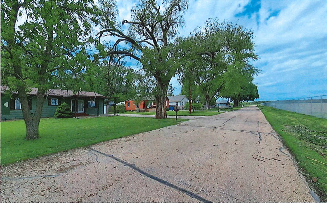
Looking North/Northwest from NE Strait Avenue 200 feet North of NE Belmont Intersection
