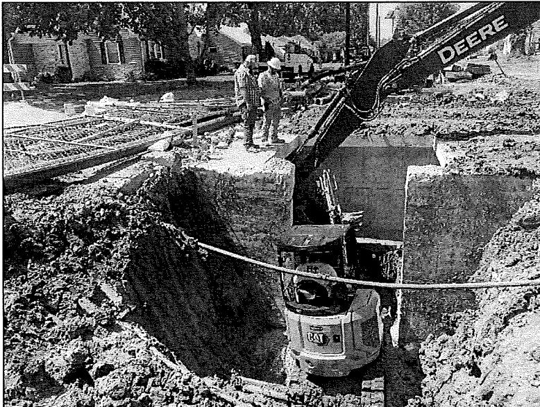
A utility contractor is placing a utility line underneath a concrete stormwater culvert that runs perpendicular underneath SW 12<sup>th</sup> St. at SW Cambridge Ave.
