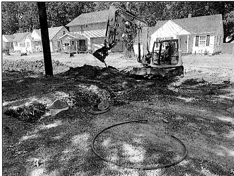
New water service lines from the main to the meter are being placed near SW 12<sup>th</sup> St. and SW Cambridge Ave.
