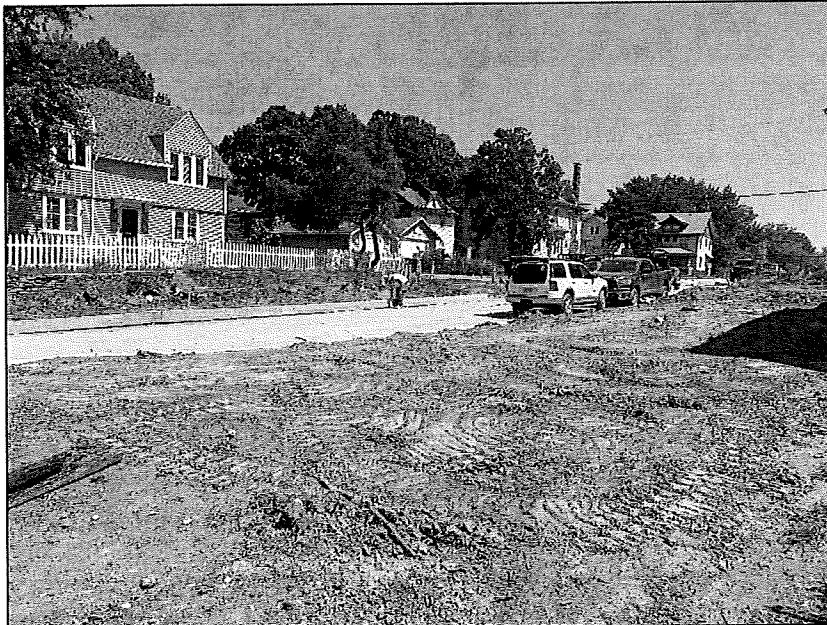
Curb forms are being placed on 12<sup>th</sup> St. just east of the Boswell Ave. intersection. Once the curbs are in place, base lifts of asphalt will be placed.
