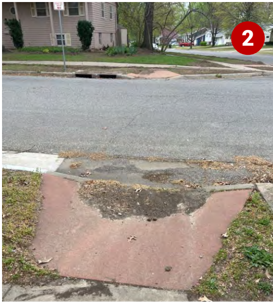
Curb ramps obstructed, not ADA compliant at SW 25 th Terrace and SW Belle Avenue
