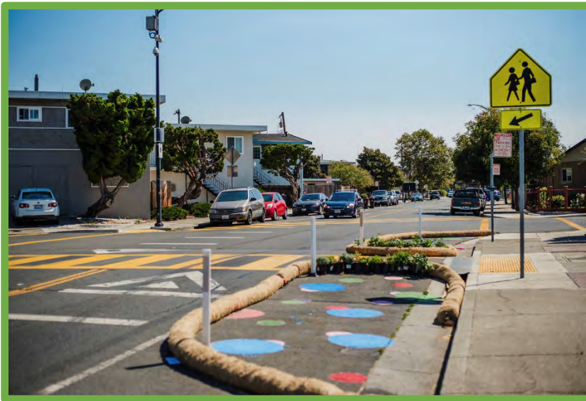
Temporary curb extension comprised of straw wattles and potted plants
