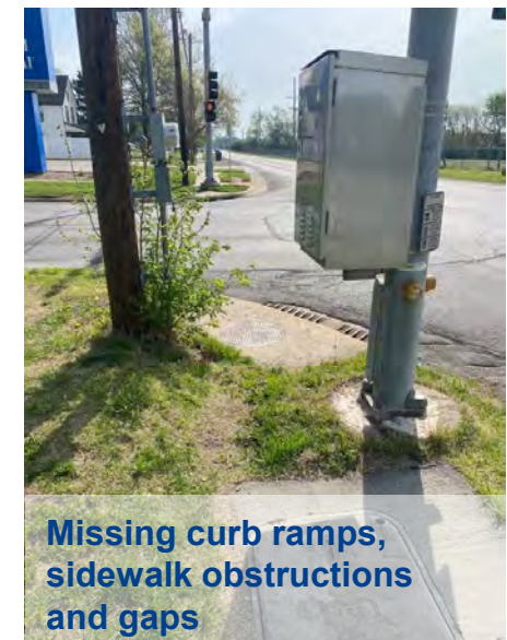
Sidewalk in poor condition, missing curb ramp and crosswalk marking
