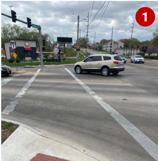
Faded markings and inadequate crossing time at SW Gage Boulevard and W 29 th Street intersections
