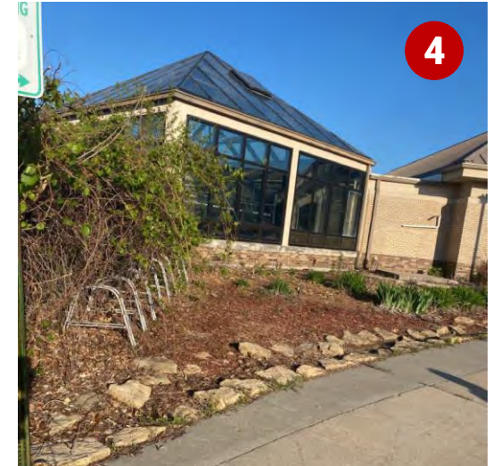
Bike rack in poor condition at school driveway
