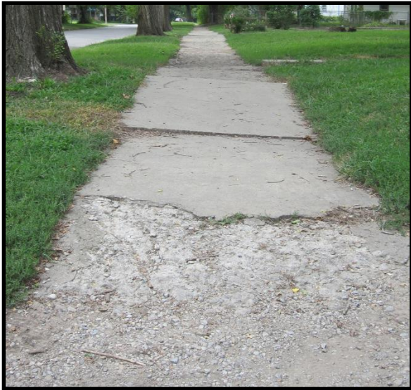
Crumbling and raised sidewalk along NE Monroe St., less than a block away from Quincy Elementary
