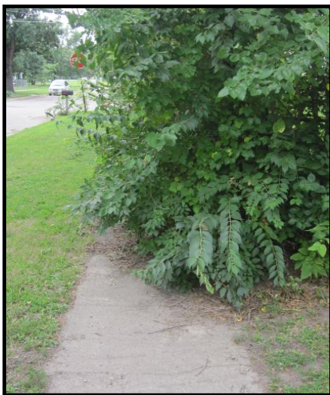
Overgrown weeds covering sidewalk on NW Harrison St., N of Paramore St.
