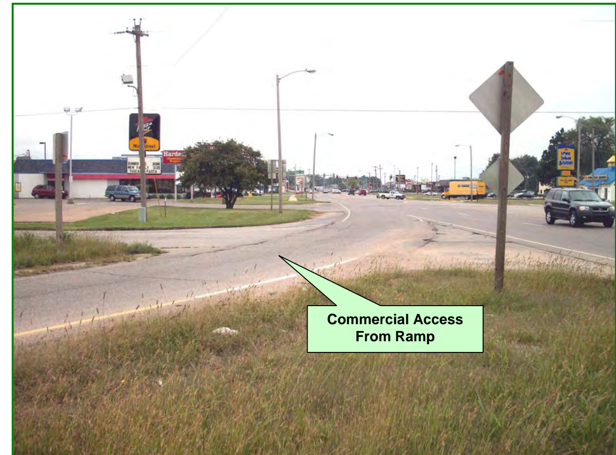
Figure 3.7 US-24 Eastbound On-Ramp From Topeka Boulevard
