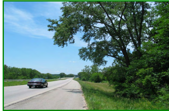
Figure 6.7: US-24 Looking West Near Calhoun Bluffs
