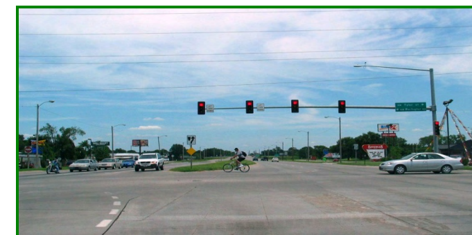
Figure 6.6: US-24 at Tyler/Rochester Looking East
