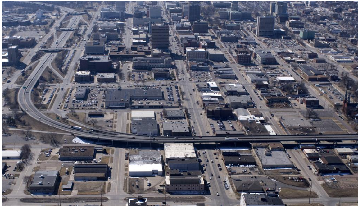
I-70 Polk-Quincy Viaduct in Topeka, KS looking south
