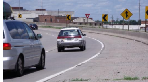
WB I-70 curve near 3 rd Street
