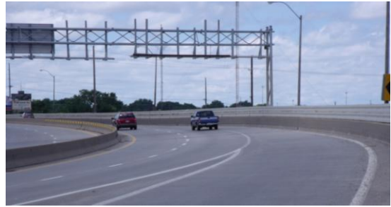
WB I-70 on-ramp from 3 rd Street
