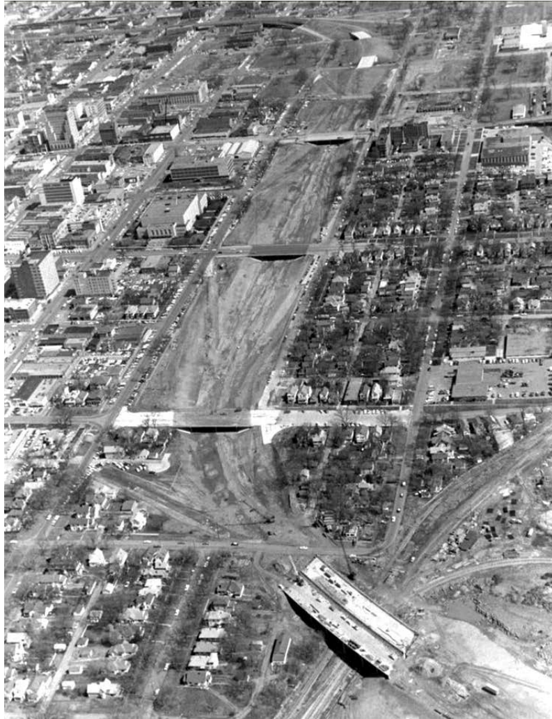
Construction of I-70 through Downtown Topeka, KS looking north towards the Polk-Quincy Viaduct (1964, KDOT)
