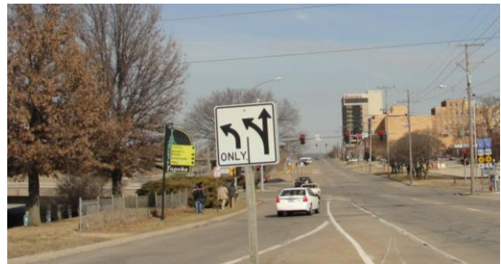
WB I-70 off-ramp approaching 8 th Avenue
