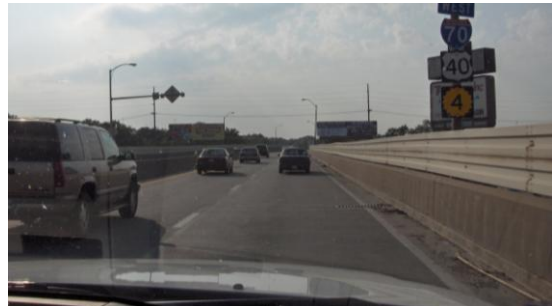
WB I-70 on the Polk-Quincy Viaduct
