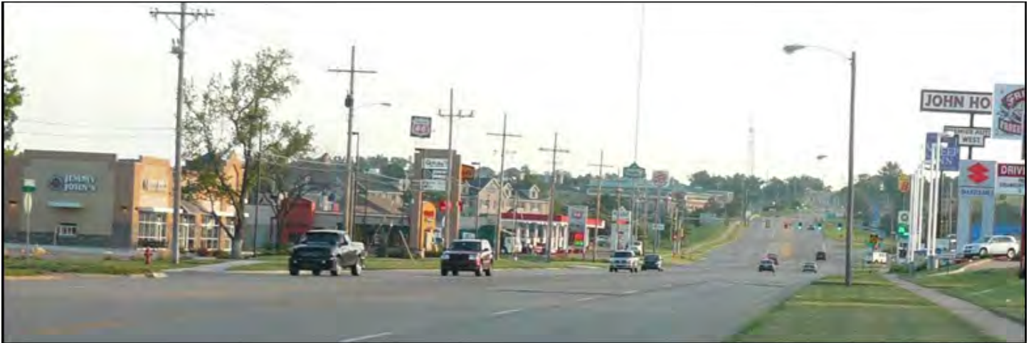
Overhead Power Lines on Wanamaker Avenue
