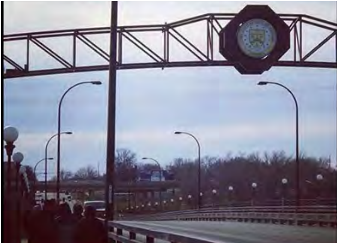
Topeka Boulevard Bridge
