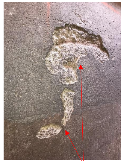
Spalled concrete slab
