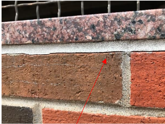
Failed sealant
