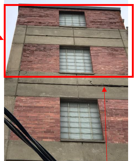
Spalled face of concrete spandrel beam. Spall should be removed for safety concerns
