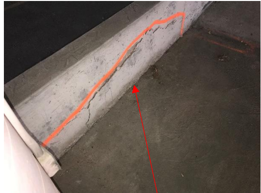
Spalled face of concrete wall
