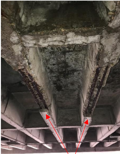
Deteriorating concrete and reinforcing steel joint stem
