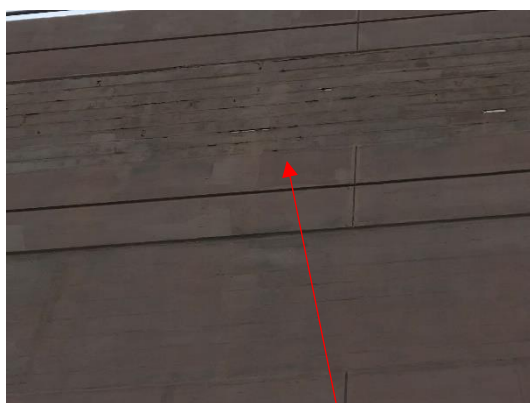
Spalled face of concrete spandrel beam
