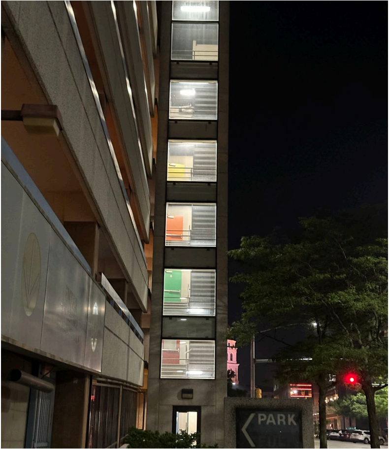
Stairwell Lighting Upgrades and LS Lighting.
