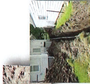
Replacement of Collapsed Sewer Line
